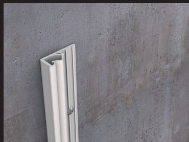
Installation of the fixing profile
